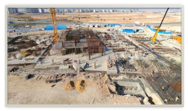
The raft foundations have been laid for all five towers and work is under way on the first storey (Hill International)
