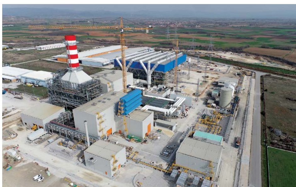
Komotini combined cycle gas turbine power plant
