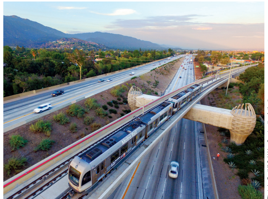
Foothill Gold Line Extension, CA.
