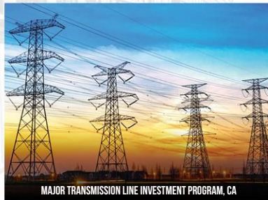
MAJOR TRANSMISSION LINE INVESTMENT PROGRAM, CA
