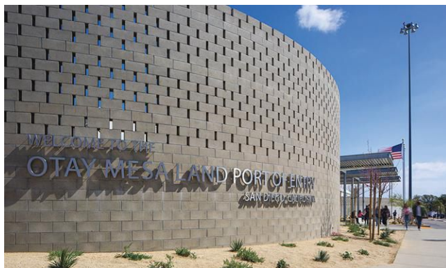
In recognition of the team’s success, the Otay Mesa LPOE project received Engineering News-Record California’s 2024 Award of Merit-Government/Public Building.
