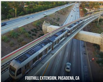
FOOTHILL EXTENSION, PASADENA, CA
